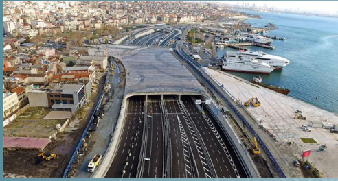
EurAsia Tunnel in Istanbul, Turkey
