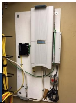
Remote Unit Installation
