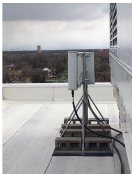
Donor Antenna Installation
